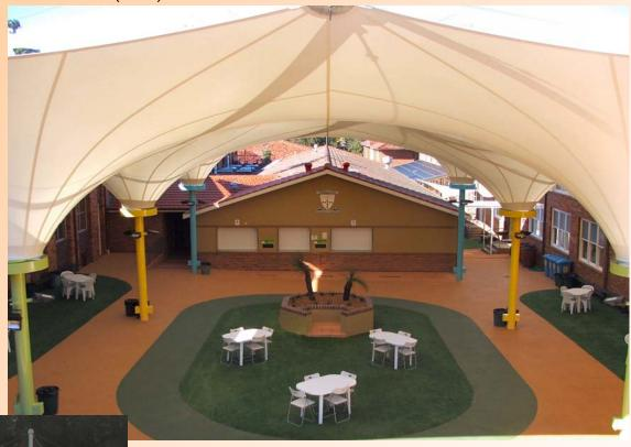
A quadrangle is totally transformed using this massive inverted conical canopy comprising 6 conical structures. The structure is completely free standing and independent, transferring no loads to existing buildings in close proximity. Water drains through the columns and into an underground stormwater system.
